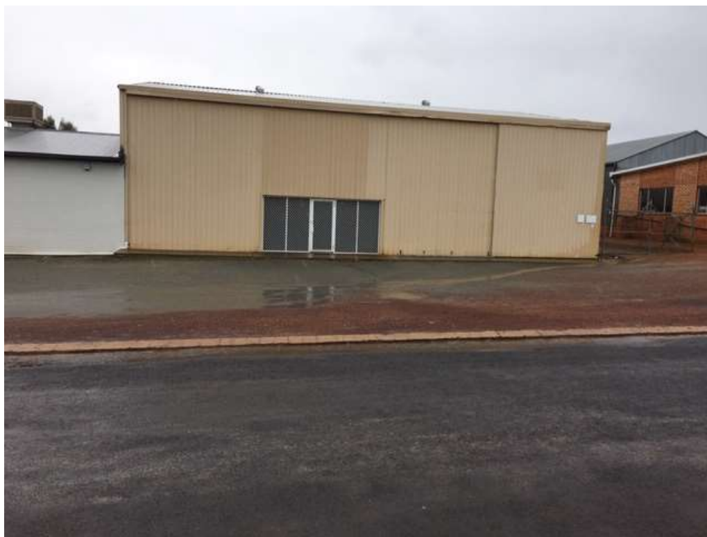
Photo 3: Generous on-site parking
