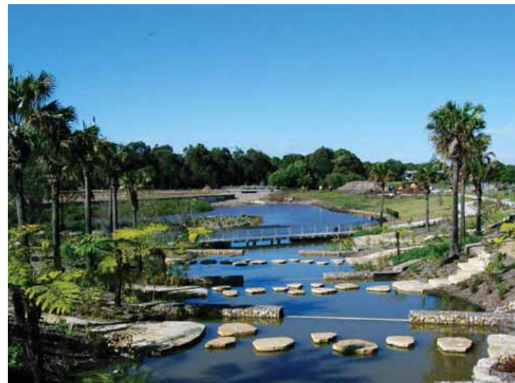
WEIRS DISPERSING WATER FLOW
