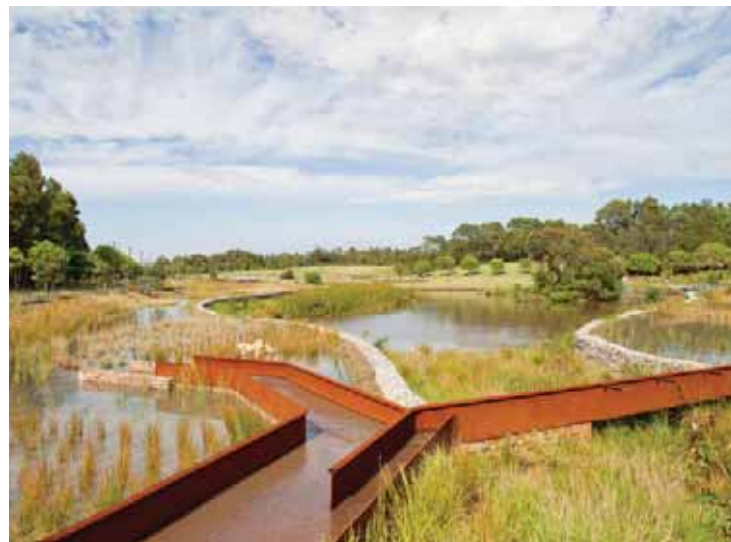
STORM WATER TREATMENT POOLS
