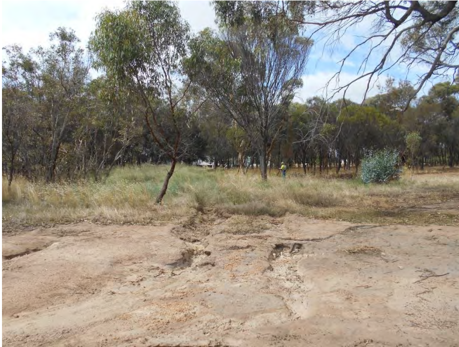
Plate 8: 4WD Access contributing to erosion issues
