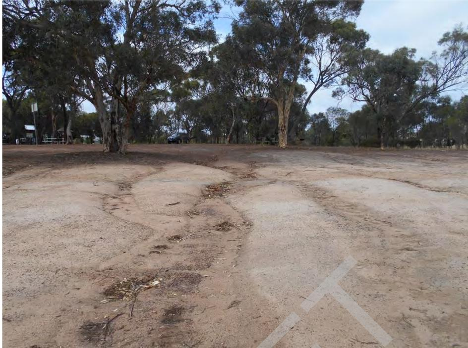
Plate 5: Erosion of banks of Railway Dam
