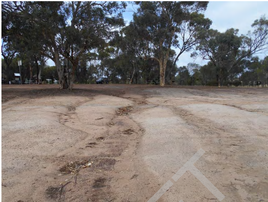
Plate 5: Erosion of banks of Railway Dam
