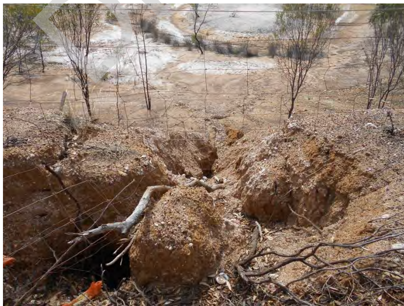
Plate 1: Erosion on banks of Archibald Park
