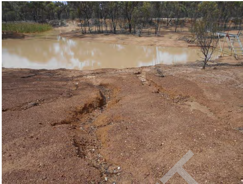
Plate 2: Erosion at Archibald Park
