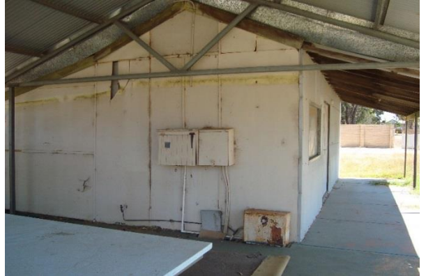
Tennis Court Club Rooms
