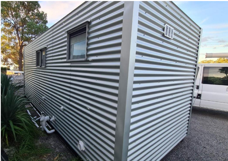
Photo 2 – Rear and Left Side Elevation
