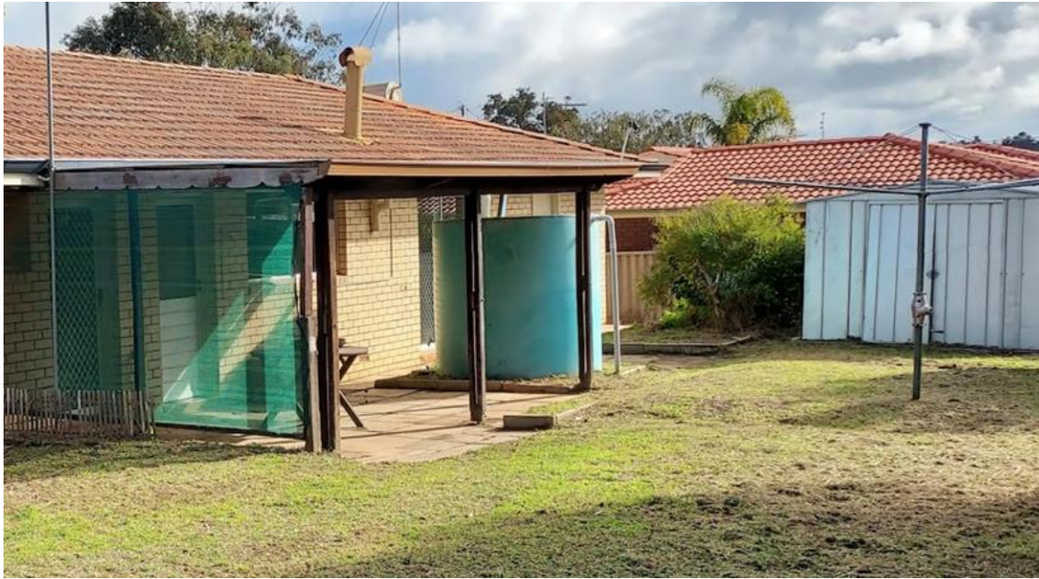
Figure 5 – Similar roof profile and materials already evident on the main house
