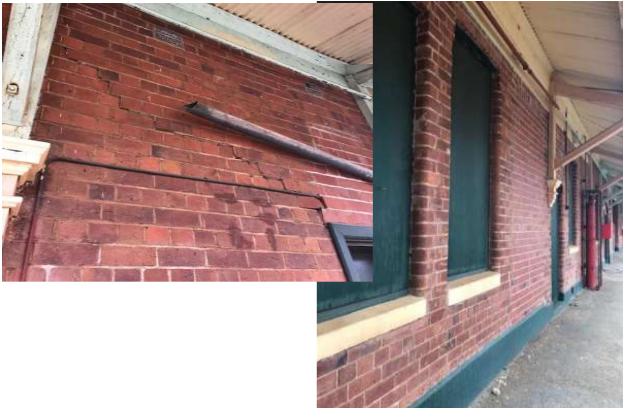
Photo 32 Narrogin Railway Station View south on the west wall.
