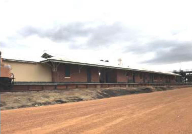
Photo 8 Narrogin Railway Station View looking northwest in Pioneer Drive showing carpark area.
