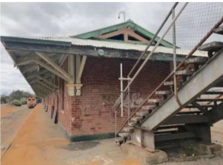
Photo 12 Narrogin Railway Station View of the north end looking south down the east side.
