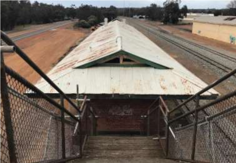
Photo 11 Narrogin Railway Station View looking south from the stairs off the pedestrian overpass.
