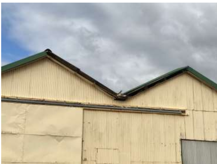
Photos 87-89 Goods Shed . North elevation showing the loading ramp; view looking to southeast showing the west side; and, detail of the north gable and wall.
