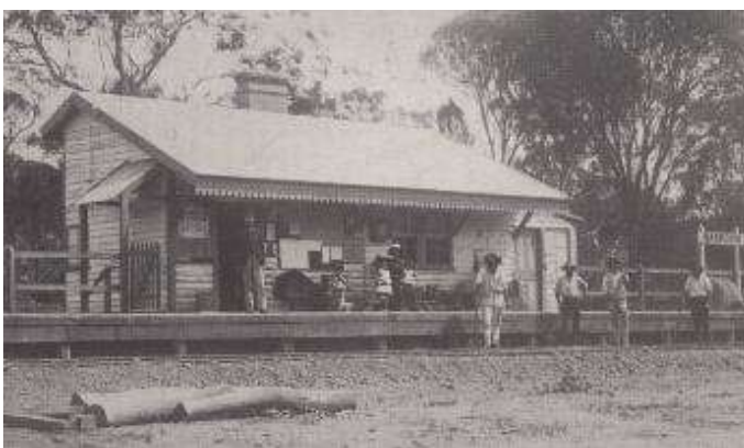
c.1889 original Narrogin Railway Station building.
