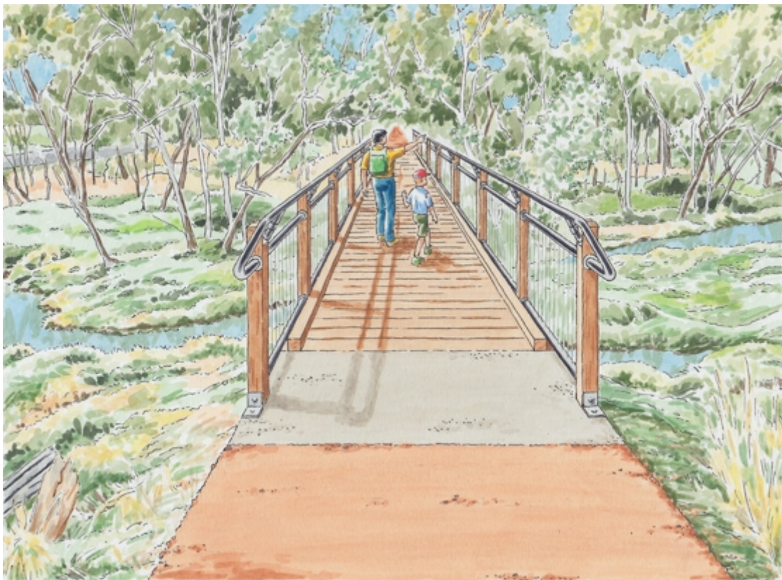
The refurbished bridge includes new decking and handrails, suitable for cycling and walking.
