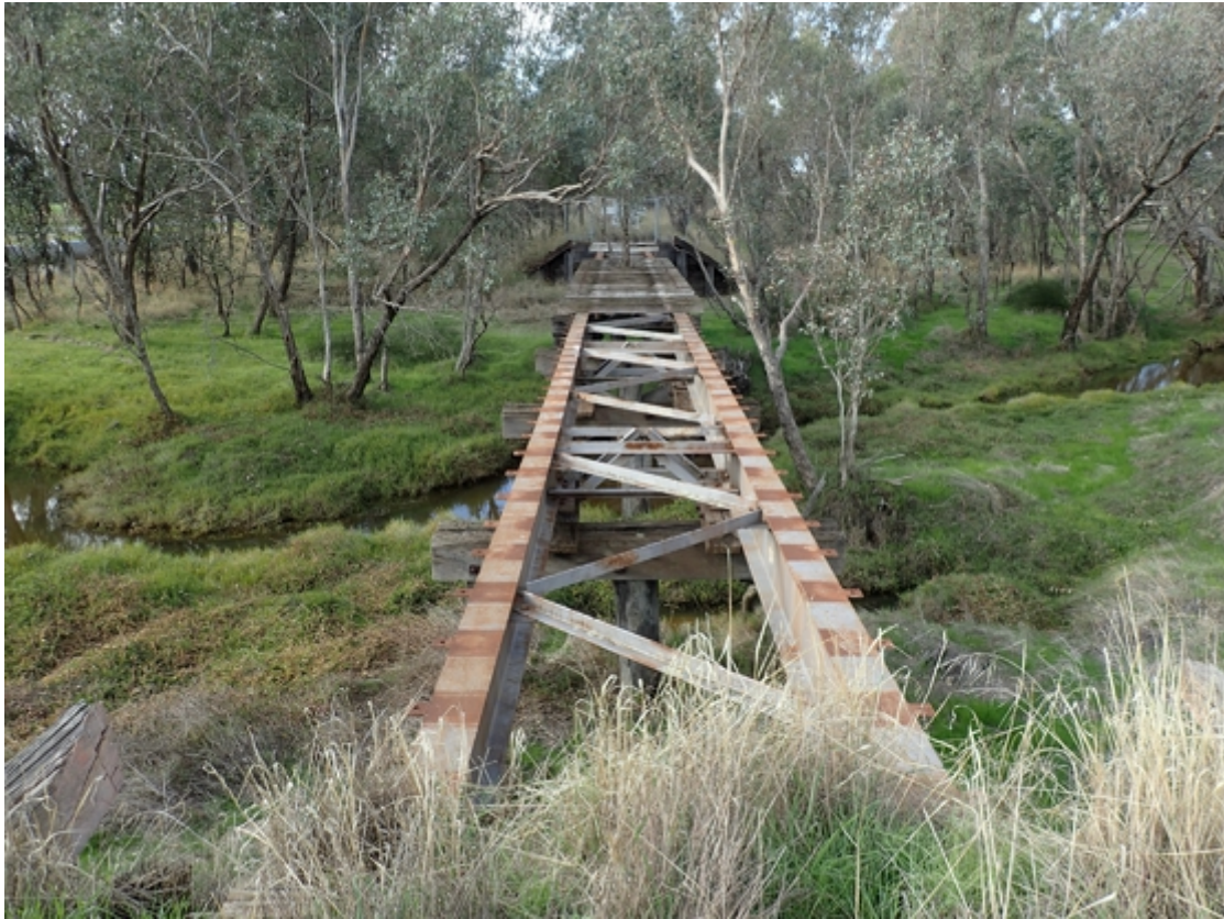
The partly dismantled railway bridge over the Williams River floodplain.
