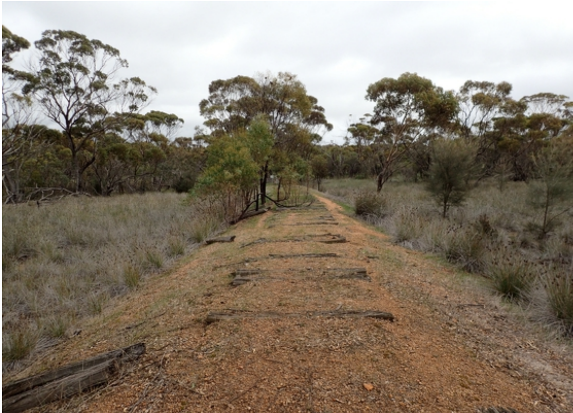
Most, but not all, of the old railway sleepers have been removed from the disused railway.
