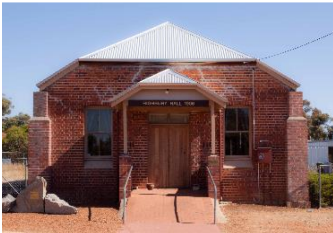
HIGHBURY DISTRICT HALL 2013
